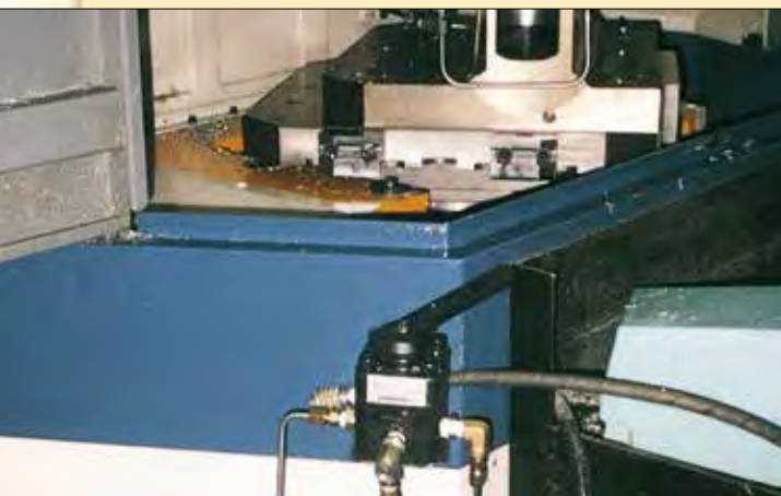
■ Enerpac VC-4 manual valves mounted to control hydraulic circuit on pallet fixture
