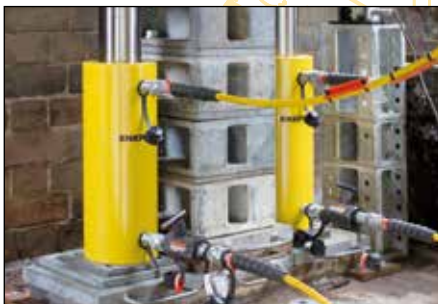
Bridge lifting and launching
