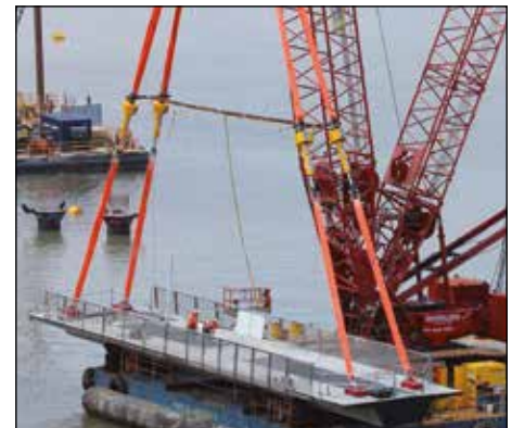
▼ SyncHoist lifts and positions Brisbane Riverwalk concrete girders
