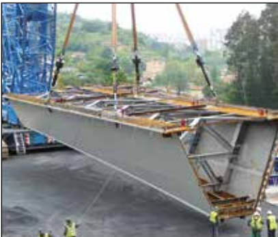
▼ Bridge segments are hoisted from the ground, being positioned with a 4-point SyncHoist system with fully monitored cylinders.
