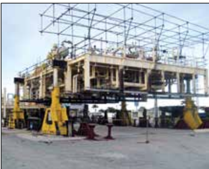
Assembling an Offshore Platform Oil Rig Module
