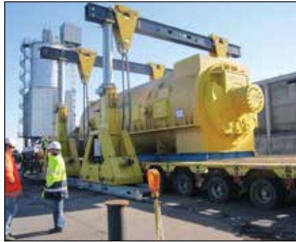
Turbine Lift and Load-in at Shipping Port
