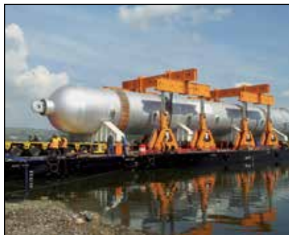
Offloading a 1300 Ton Hydrocracker
