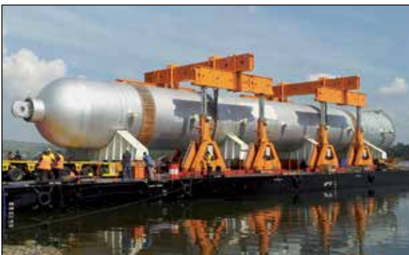
◀ Two SBL1100 gantry systems lifted the 1300 ton hydrocracker off the barge onto a SPMT Self-Propelled Modular Transporter.
