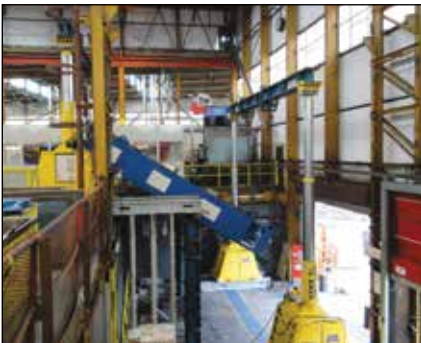
Transporting a 1200 Ton Hydraulic Press to the Second Floor with a Hydraulic Gantry
