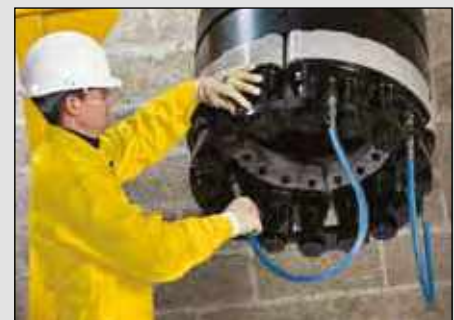
▲ Multi Stud Tensioning application.
