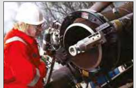
▲ Pipe cutters and weld preparation.
