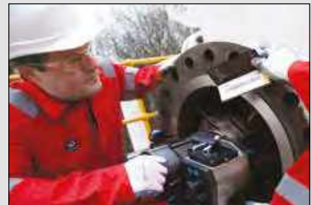
▲ Flange facing machines to ensure flange joint integrity.
