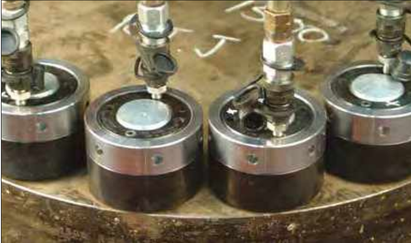
▲ Tensioning with hydraulic nuts.
