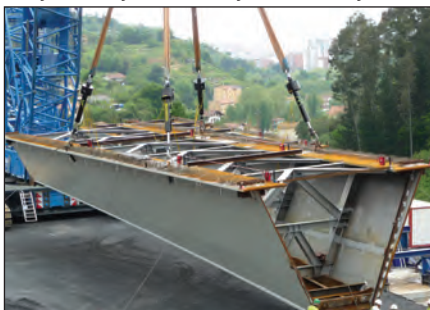
▼ Bridge segments are hoisted from the ground, being positioned with a 4-point SyncHoist system with fully monitored cylinders.
