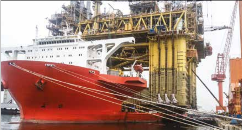
▲ The superlifting and launch of a 43.000-ton floating oil production system in Malaysia for the Gumusut-Kakap offshore field has set high benchmarks for safety through its use of sophisticated EVO-Series synchronous hydraulics to lift, balance, weigh and smoothly launch massive resource structures.
