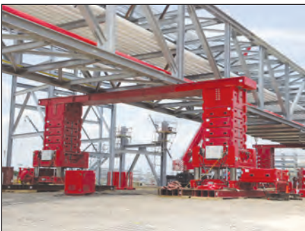
▼ Lifting an oil and gas pipe module
