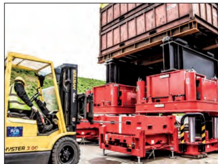
▼ A load is lifted in increments as barrels are slid into the system, lifted, and stacked; forming 'lifting towers'.
